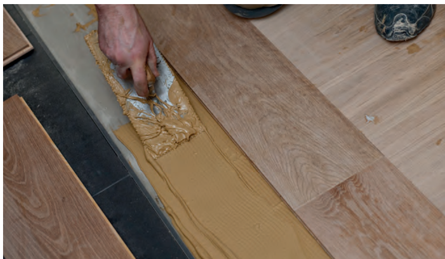
A specialist wood adhesive must be used during installation
