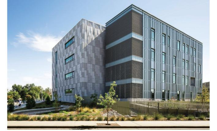
The exterior of the building boasts mechanically attached Sierra White™ granite in a vertical, basket-weave pattern.
