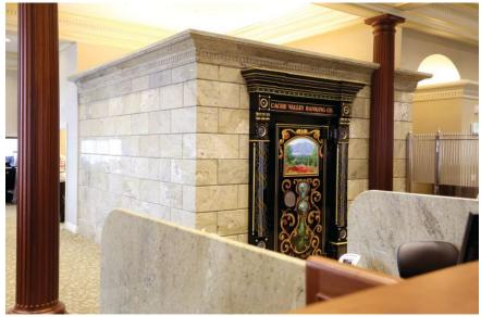
The motif used on the top of the vault, creating a multimember crown molding complete with dentil mold, was a bit of a challenge as it was something that the fabricator never contemplated prior to this project.
